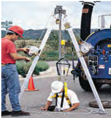
Tripod used for safe entry
