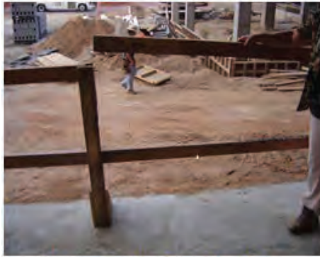
Removable Guardrail at second Floor
