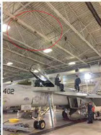
Overhead Beam Strap with Self Retracting Lanyard
