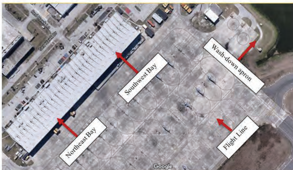
Figure 2. The northeast and southwest bays of Hangar 1552, the wash-down apron, and flight line at Naval Station Mayport.
