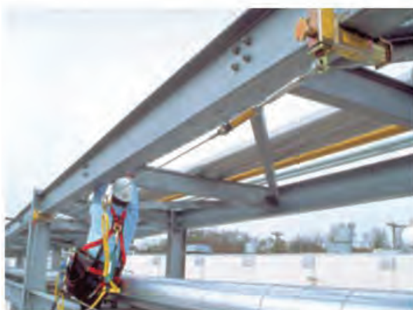
Mobile Attachment Device for moving between intermediate anchorages
