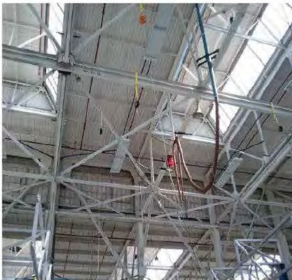
Overhead Beam Strap with Self Retracting Lanyard
