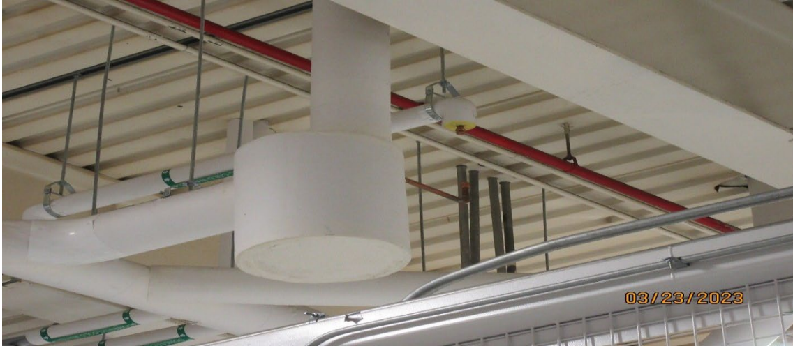
Picture 6. Repaired Sewage Line in Building 9001
