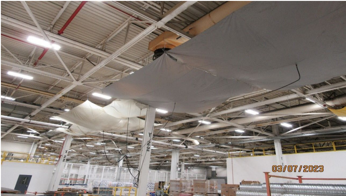
Picture 5. Umbrella tarps are used to mitigate rain from leaking onto the mechanical floors in both buildings
